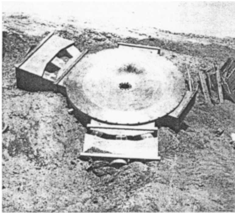
Fig. 7a—Alpha calutron chamber on its side.
